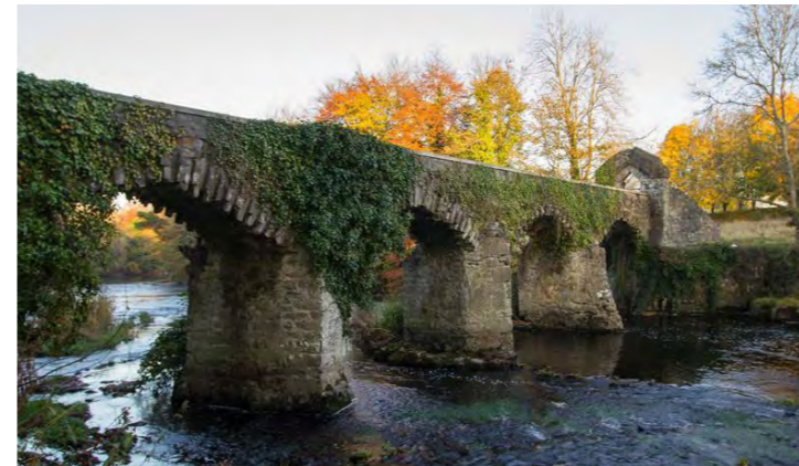
2. Rock Bridge, Celbridge Abbey, 1725-1775
