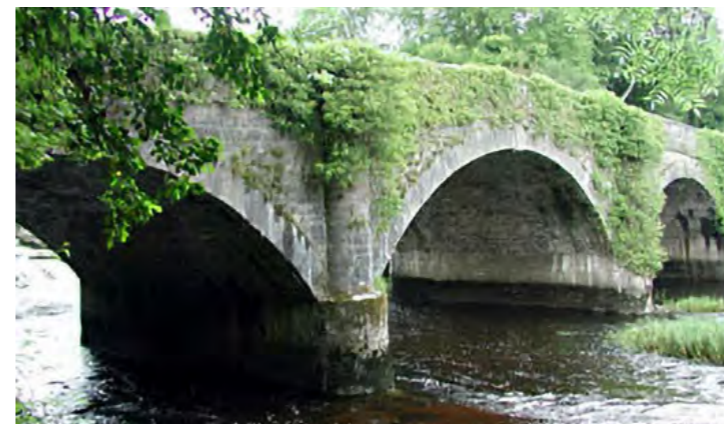
4. Straffan Bridge, Straffan, 1830-1870
