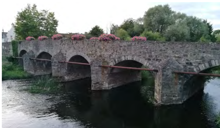
3. Celbridge Bridge, Celbridge, 1800-1820
