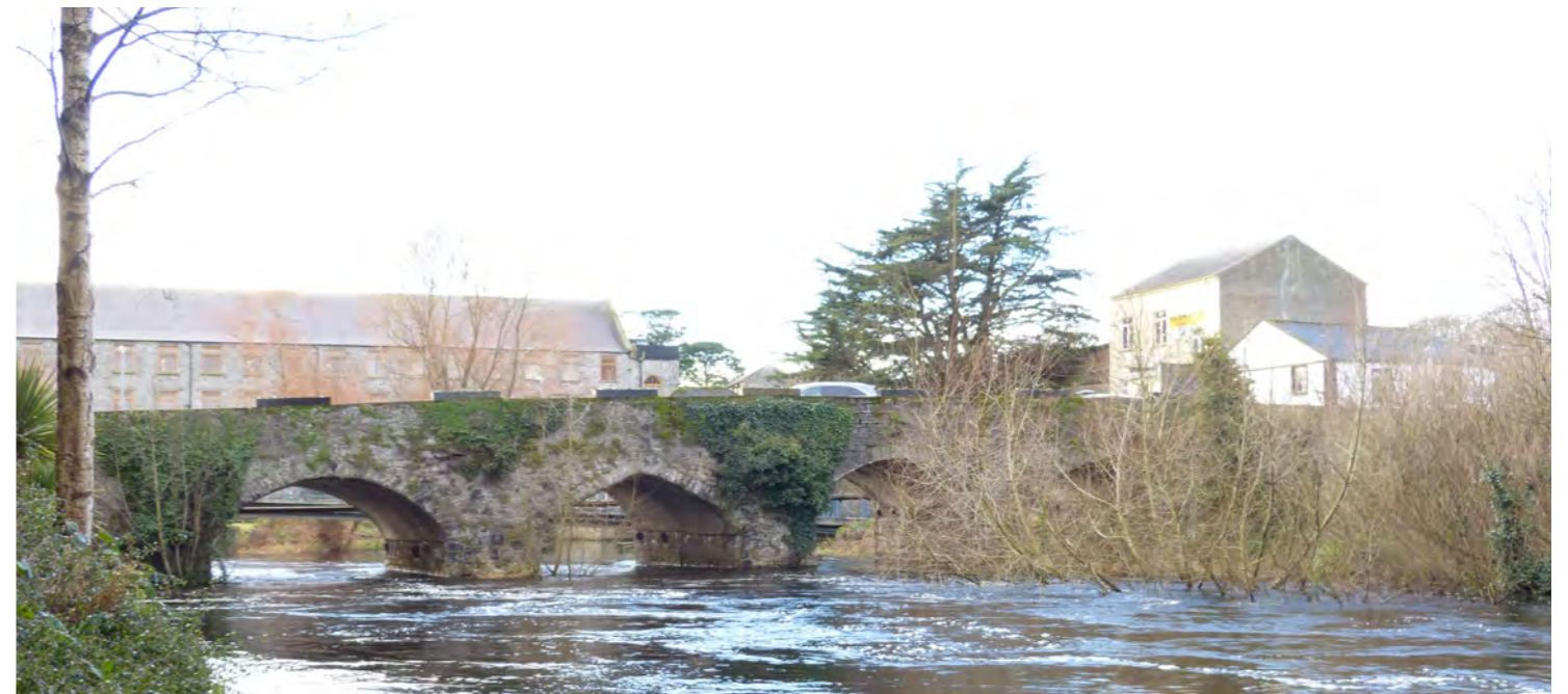
North Side Celbridge Bridge, Current
